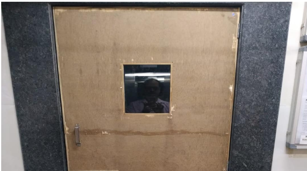
Duct Door: Door has been fixed in from of the duct giving a neat look. It will soon be painted.
